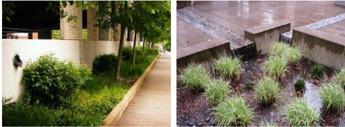
Figure 4.24-1: Various Stormwater Planters
