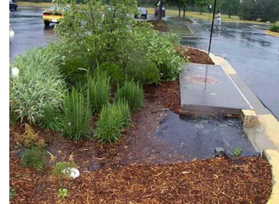
Middle Right: Figure 4.2-4 Bioretention Area after Storm
